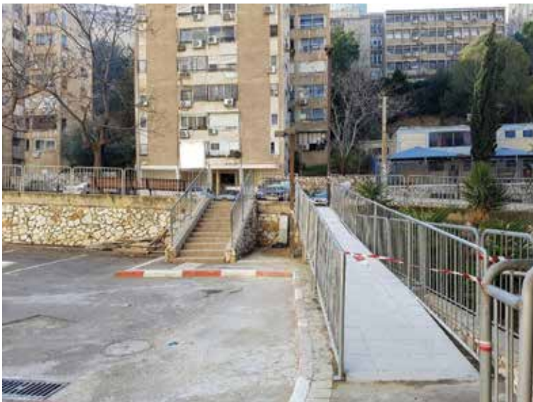
Photo 3: The ramp that was built in the housing cluster
