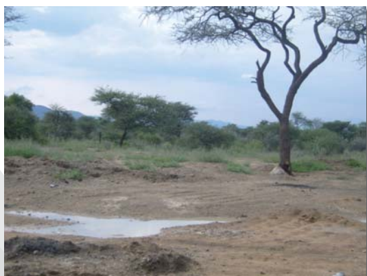
Picture showing no fence or warning signs
