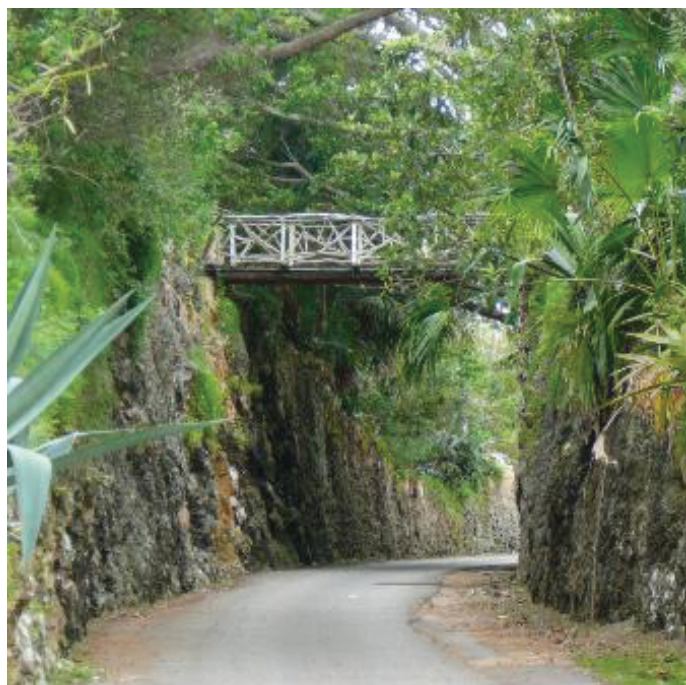
Footbridge along the railway trail in Sandys Parish
