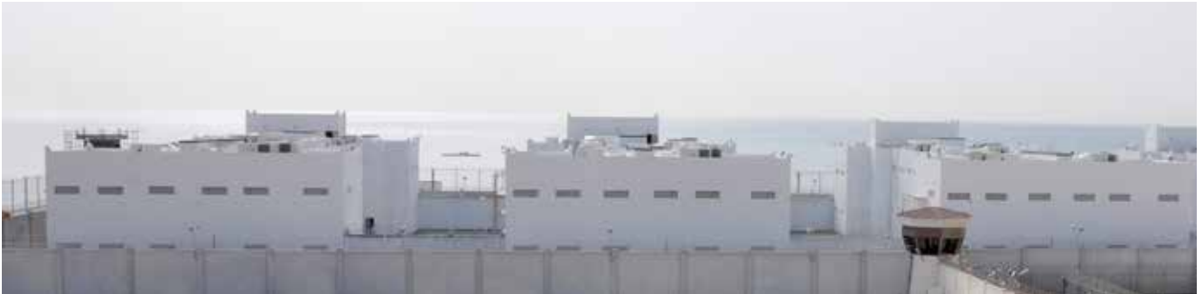
New buildings at Jau Prison to replace the old ones
