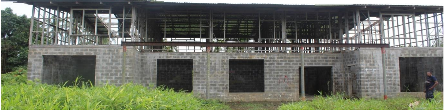
Fig 12. The incomplete District Office
