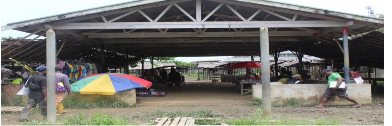
Fig 13. The incomplete Market facility
