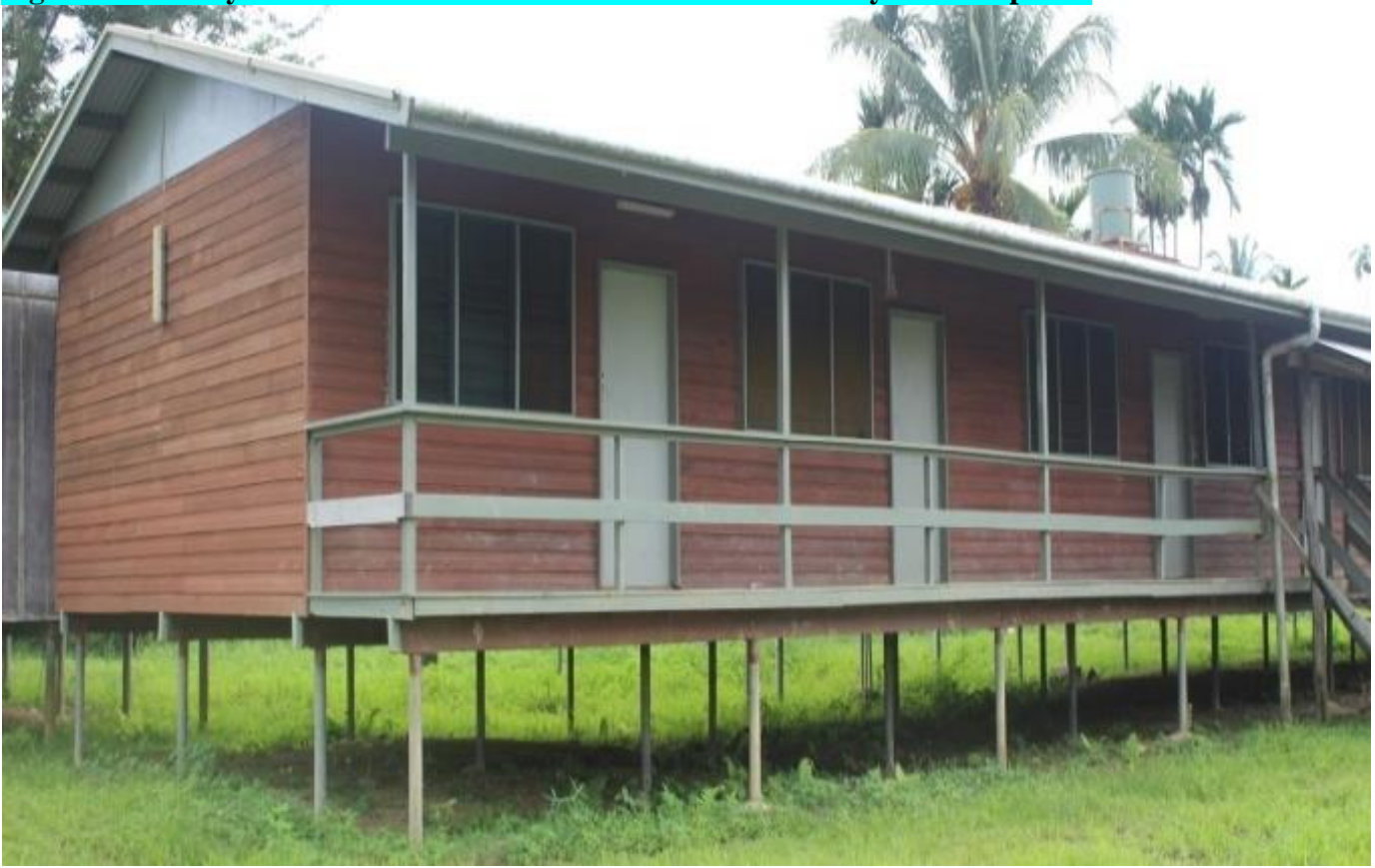
Fig 11. The newly constructed Baimuru Health Centre which is yet to be opened
