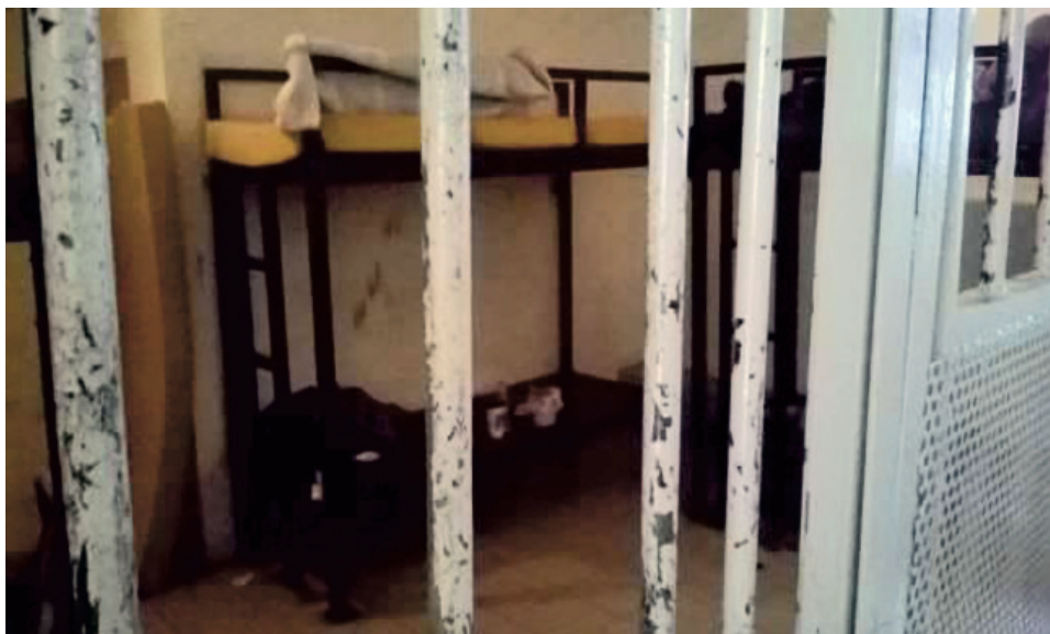
Larissa Security Department cells - inspection on 1/10/19
