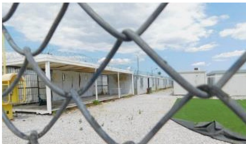
Amygdaleza Pre-removal Detention Center (Attica) - inspection on 18/7/19
