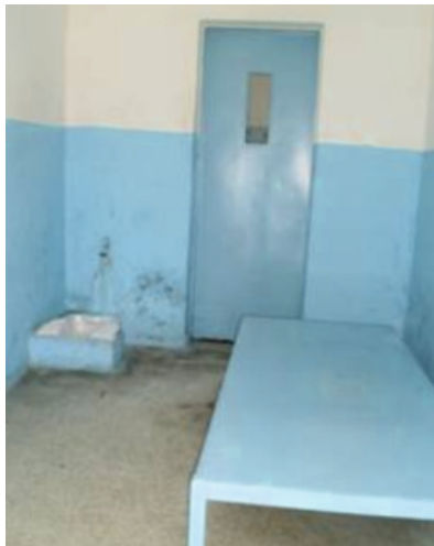
Larissa detention facility - inspection 30/9-1/10/19
