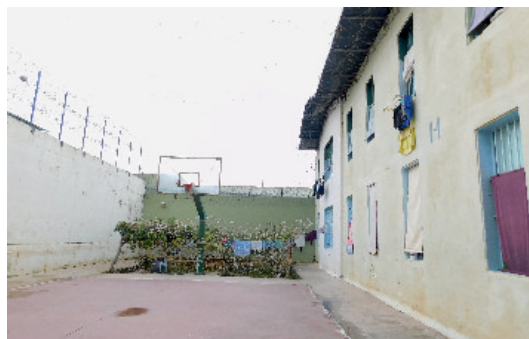
Malandrino detention facility, Fokida - inspection on 25-26/11/19
