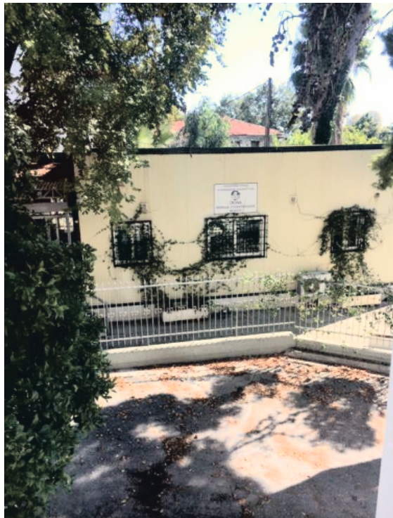
"Achillopouleio" Volos General Hospital Psychiatric Clinic - inspection on 1/10/19
