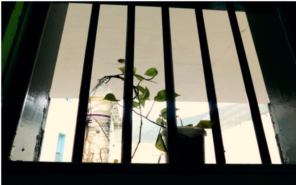
Malandrino detention facility, Fokida - inspection on 25-26/11/19
