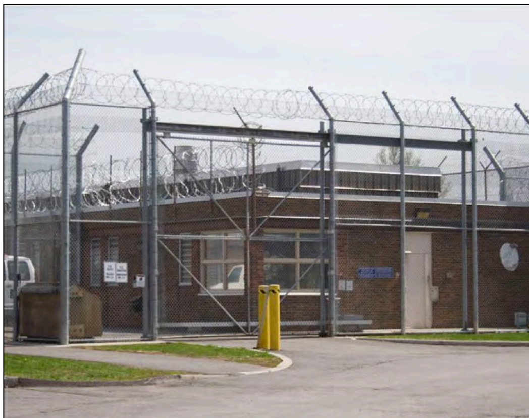
Figure 4: Ottawa Carleton Detention Centre. Photo provided by the Ottawa Citizen .
