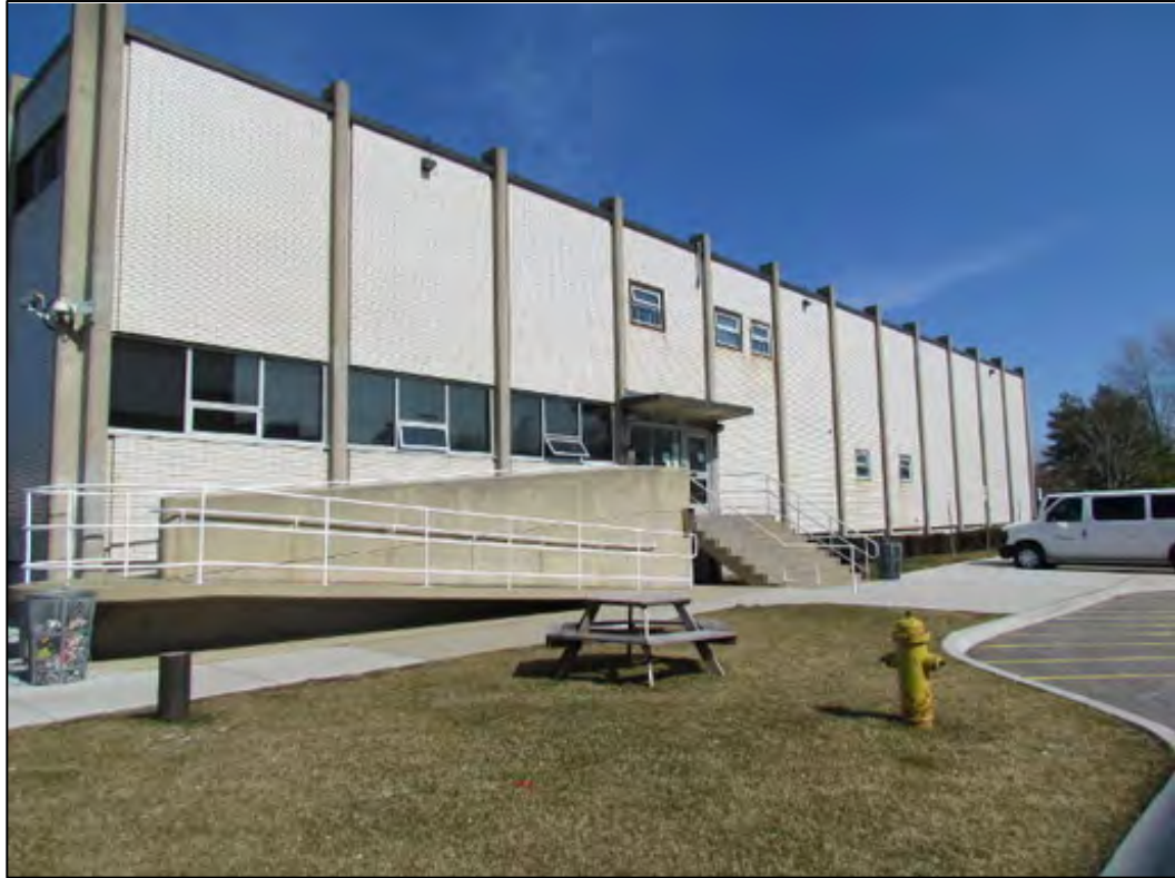
Figure 6: Sarnia Jail. Photo provided by the Sarnia Observer/Sun Media.
