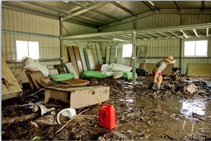
Flood damage in Grantham
